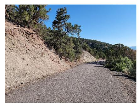
Photo 2. Steep slopes with weakly cemented surficial soils
