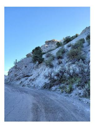
Photo 5. Steep slope with weakly cemented surficial soils
