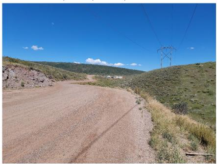
Photo 11. Rock outcrop in the potential cut section
