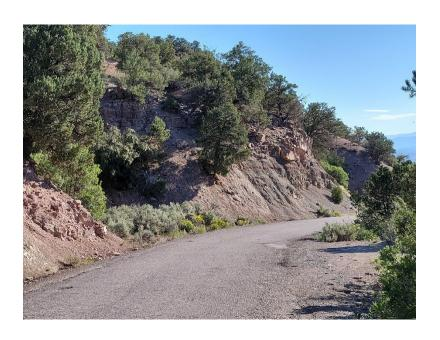
Photo 4. Rock outcrop and weakly cemented surficial soils
